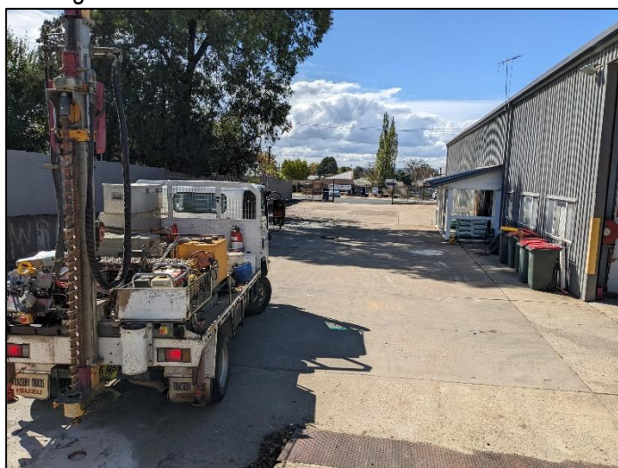
Looking north over western section of the site
