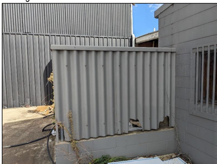
Asbestos containing fence – AEC3
